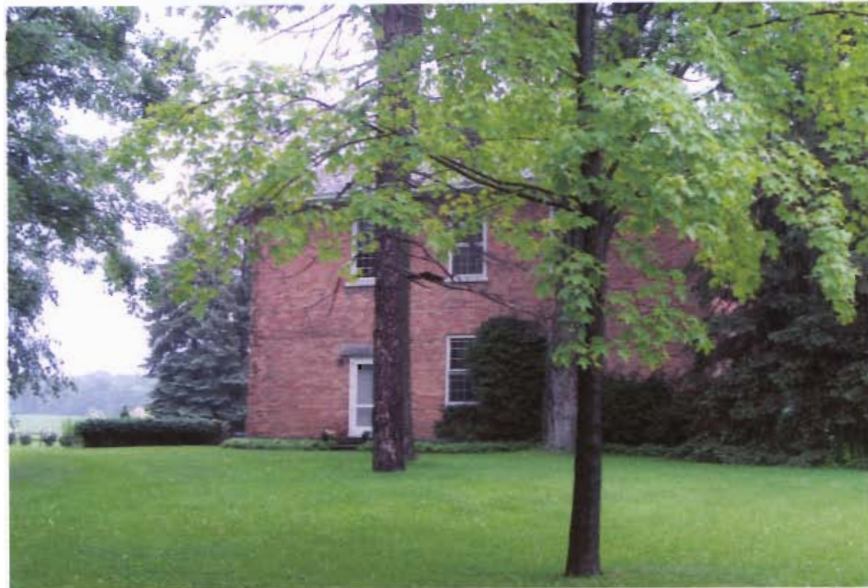
Figure 2: Brick Meeting House in Sherwood, Cayuga County 199
